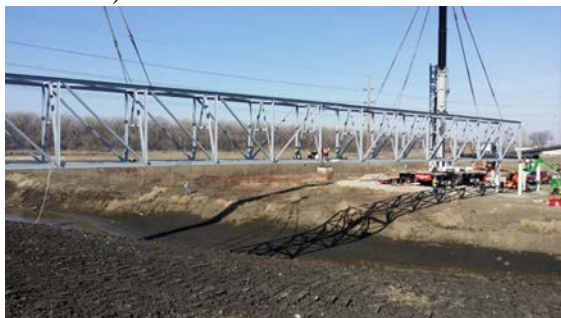
Bridge Flight on March 12, 2015. Repairs finalized in May, 2015
