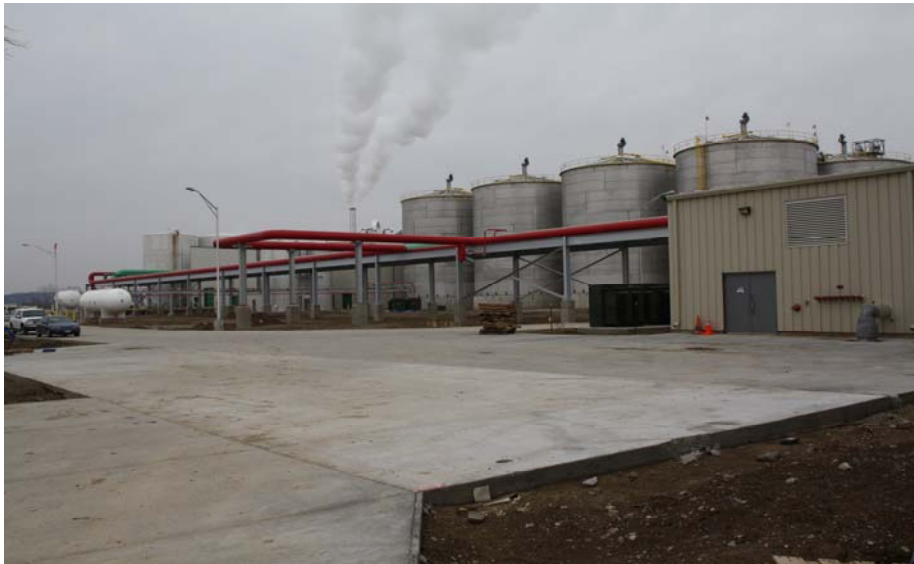
Picture 2 is looking south from the northwest corner of our site. The red pipe is the final leg of the steam line entering the plant.
