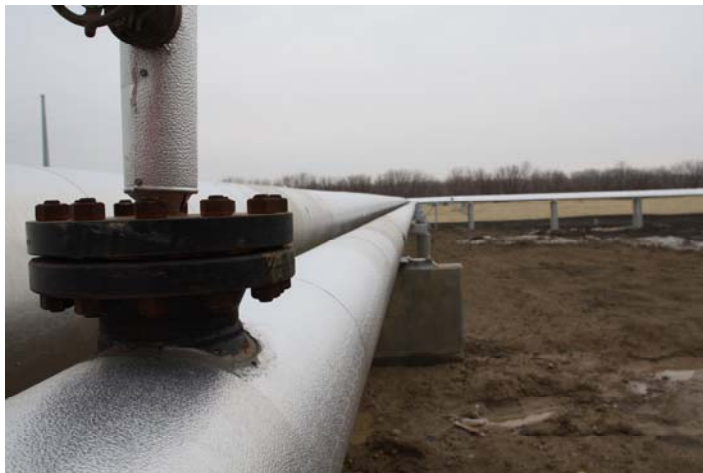
Picture 1 is looking west from the water treatment building. The pipeline veers north toward MidAm. The 14" pipe is steam coming from MidAm, the 8" is condensate returning to MidAm.
